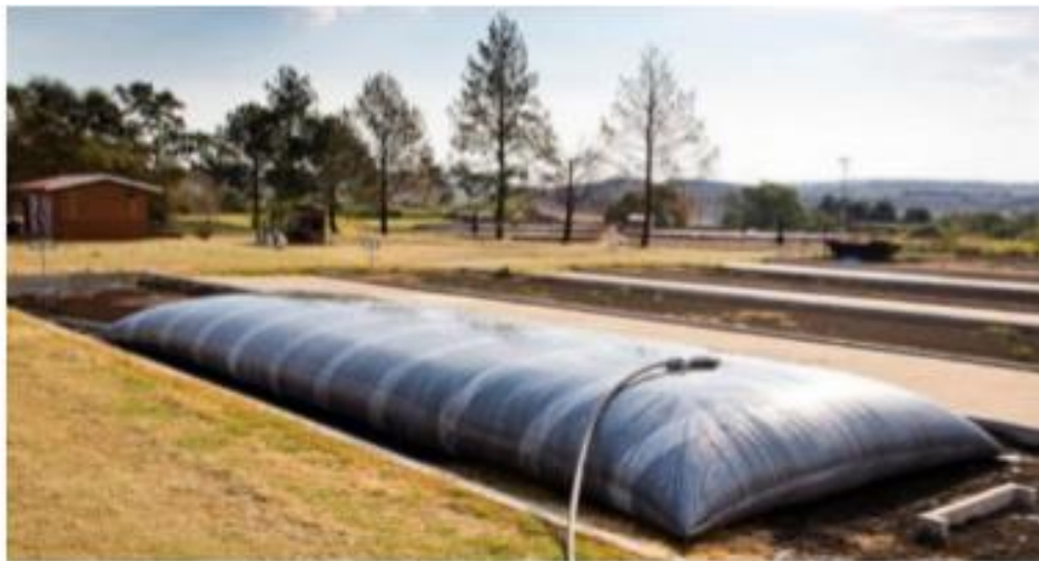
Figure 10: Schematic of Geotextile Dewatering Bags
