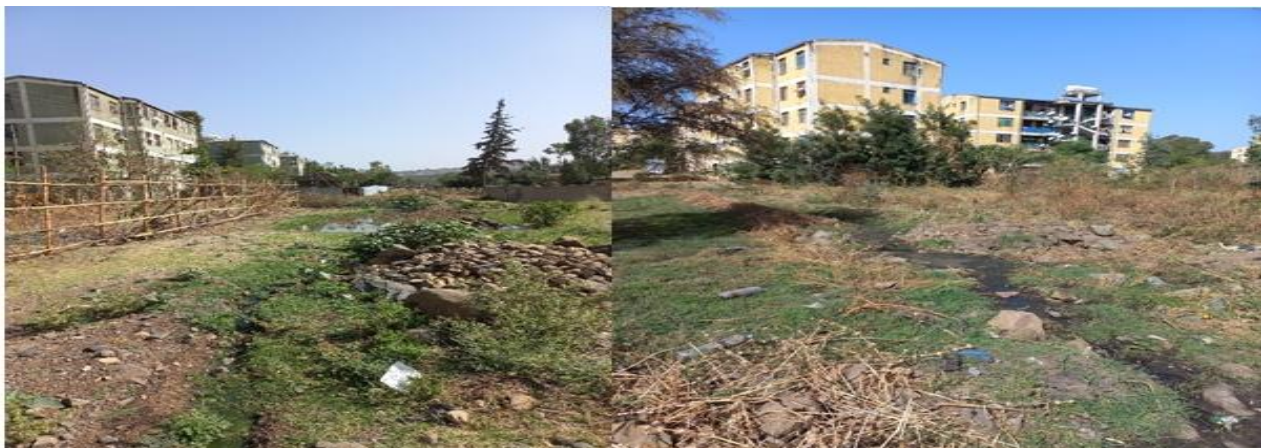
Figure 12: Improper Discharges of Wastewater Around Condominium Sites
