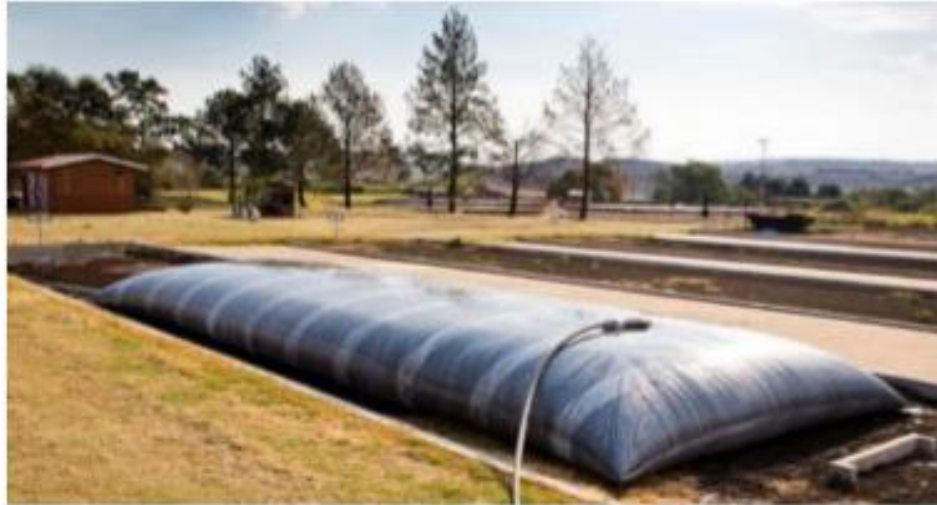
Figure 8 Schematic of Geo-textile dewatering Bags
